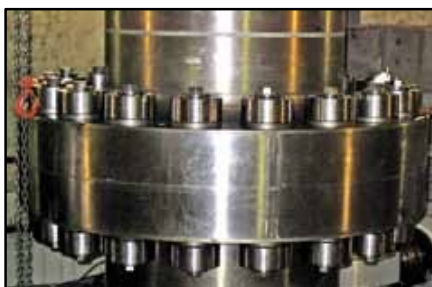
Coupling bolt installation utilizing Expansion Bolts.
