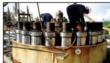
Large methanol reactor with 11" studs. Six hours with Superbolt® vs. two days with Hydraulic Tensioners.
