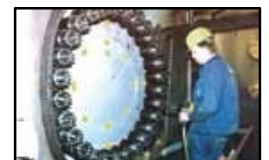
1200 MW Hydro Plant Nozzles on Pelton Turbines. Engineers were able to decrease the size of the nozzles with close spacing of the torquebolts®. Shown is the test plate being installed for hydro testing. Each 400 MW unit has five nozzles.
