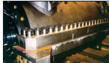
52 two inch tensioners on a centrifugal compressor were tightened in 2-1/2 hours.
