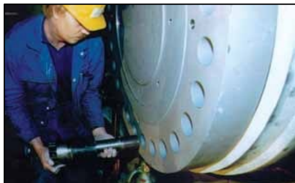
1200 MW Hydro Plant Nozzles on Pelton Turbines. Engineers were able to decrease the size of the nozzles with close spacing of the torquebolts®. Shown is the test plate being installed for hydro testing. Each 400 MW unit has five nozzles.
