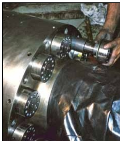
Large turbine/generator coupling. Installation 4 hours, removal 1 hour.
