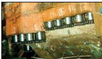
Steam turbine easily installed despite inverted position.
